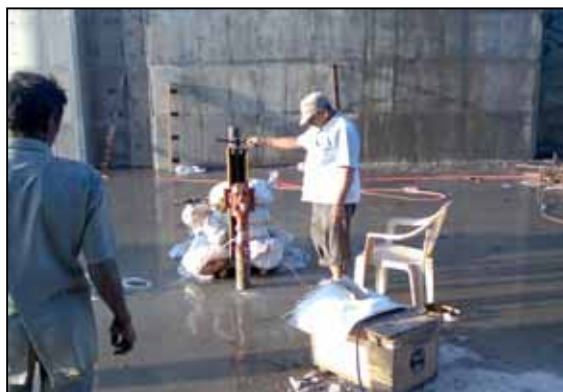
Core Drilling in Progress
