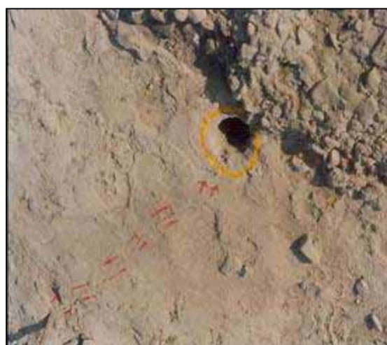
Cracks observed in body wall of M-4
