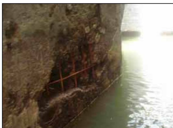
Damages in Baffle Blocks
