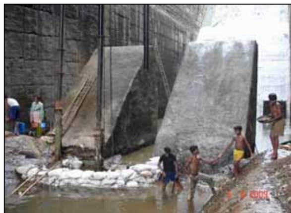
Baffle Blocks in Stilling Basin
